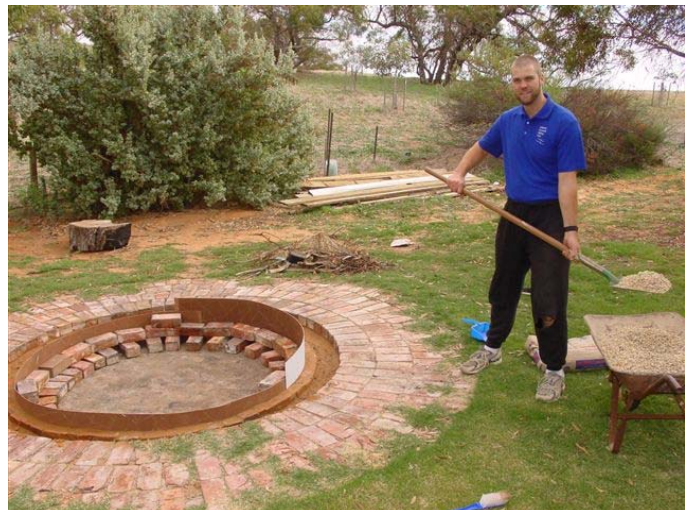
Derek Spencer concreting
